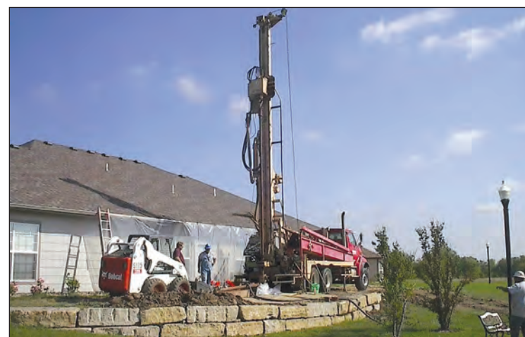
Workers plug a well that was leaking natural gas next to a long-term care center near Wichita in 2014. KANSAS CORPORATION COMMISSION
